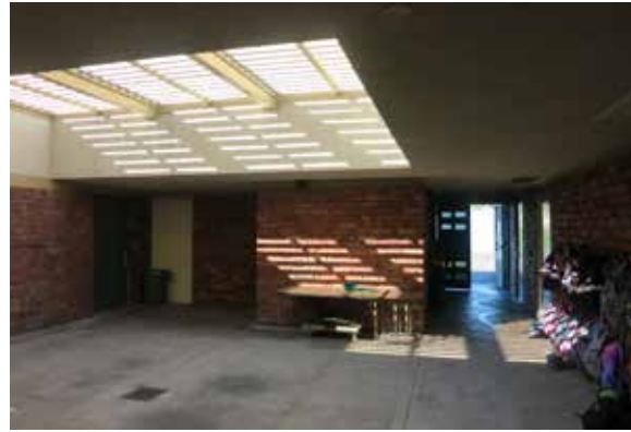
Narrow passageways between Classroom clusters and restrooms
