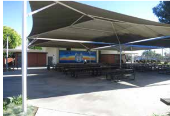
Shade structures / exterior student dining
