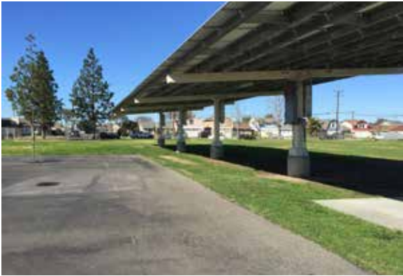
Solar shade structure at playfields
