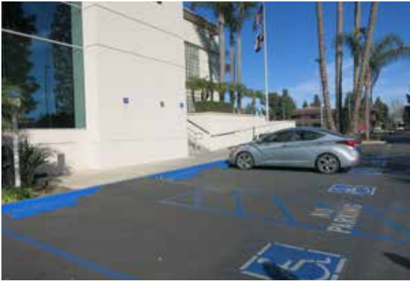
Front entry, stair, ramp and accessible stalls
