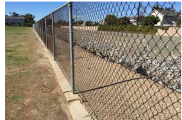
Perimeter fencing along North side of campus
