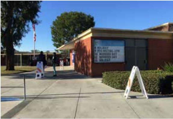
Front entrance and marquee
