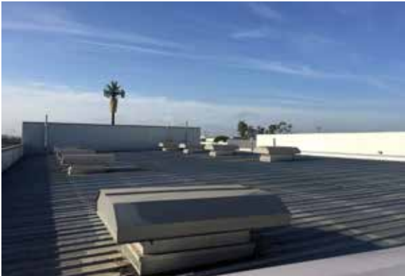
Roof at M&O warehouse
