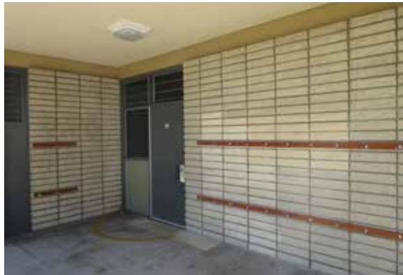
Typical exterior door
