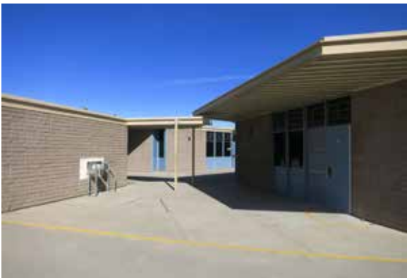
Area between classroom pods. Typical building exterior
