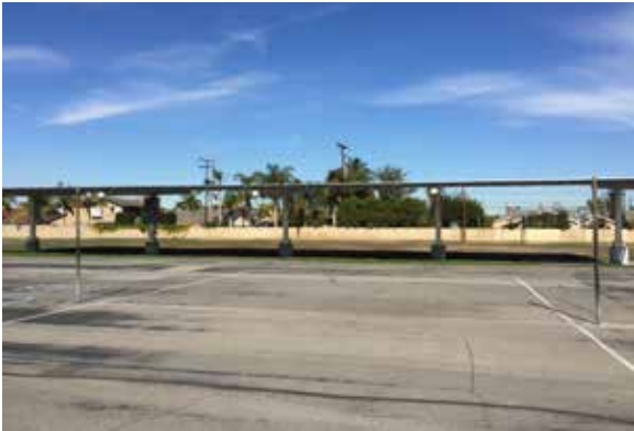
Solar shade structure
