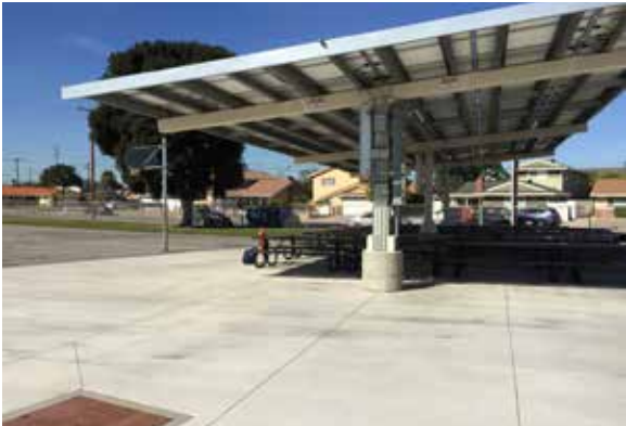
Solar shade structure/ lunch shelter
