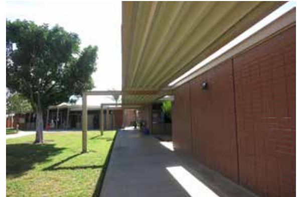
Typical covered walkway
