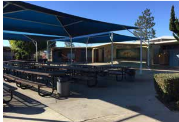
Shade structures / exterior student dining / outdoor stage
