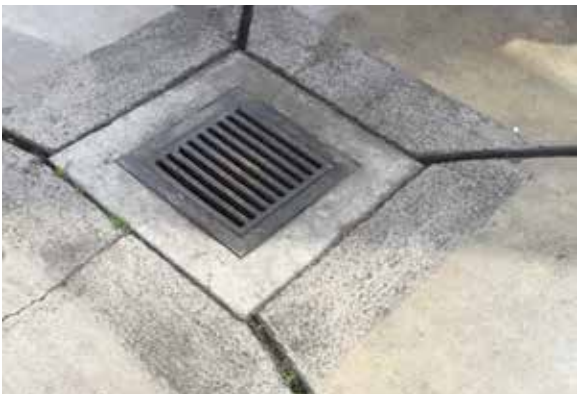
Typical exterior area drain
