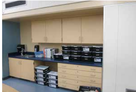
Typical interior casework
