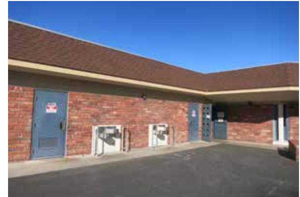
Typical exterior wall
