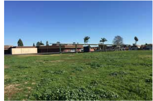
Playfield and solar shade structure
