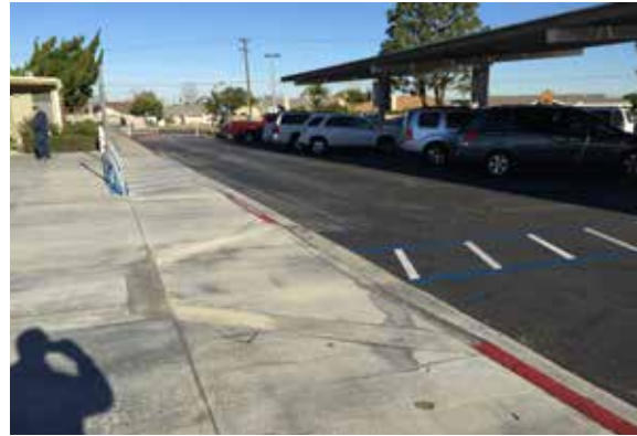
Parking and drop-off, solar shade structure
