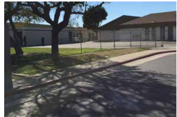
Typical chainlink fencing and gate
